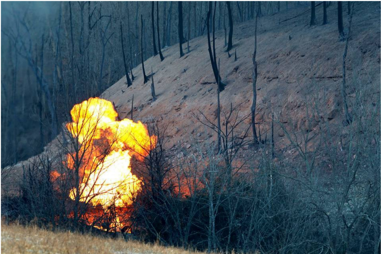
PHOTO: “Pipeline rupture in Estill County, Kentucky which was caused by overstress from land movement”: http://www.kentucky.com/news/local/crime/article44148285.html
