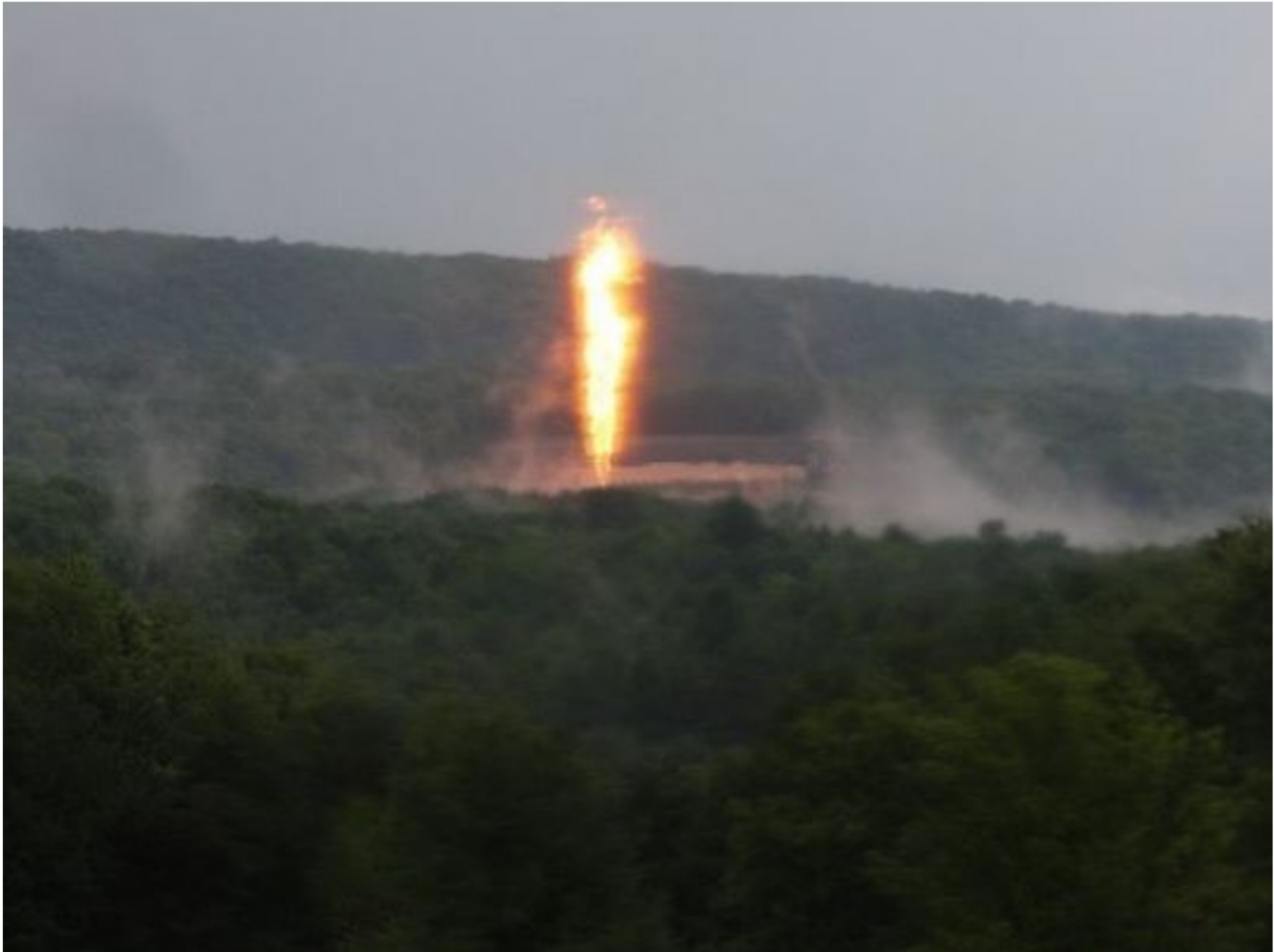
PHOTO: “In Windsor, New York, a Williams Company was venting a pipeline during a lightning storm - lightning struck the pipe and ignited the gas”:
